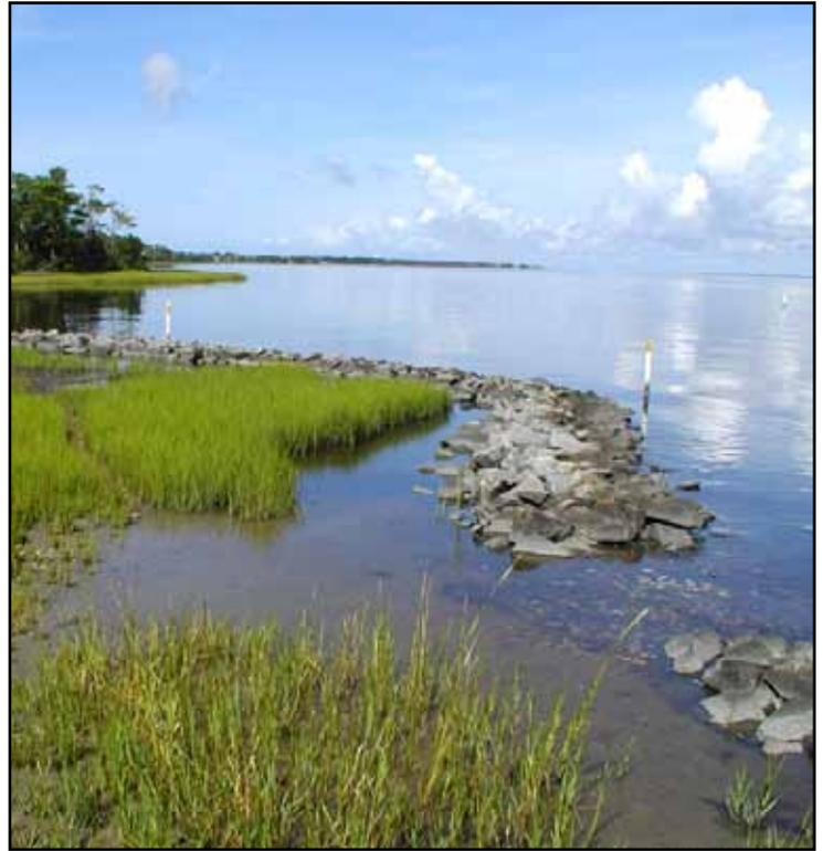
Hybrid shoreline stabilization structures that employ marsh plantings and low rock sills (to protect the vegetation) can help stabilize eroding banks. Credit: NOAA
